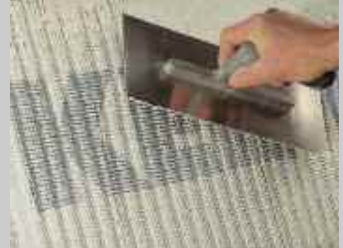
2 Optional placement of mesh
