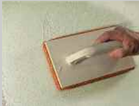
4 Rubbing in with coarse sponge float
